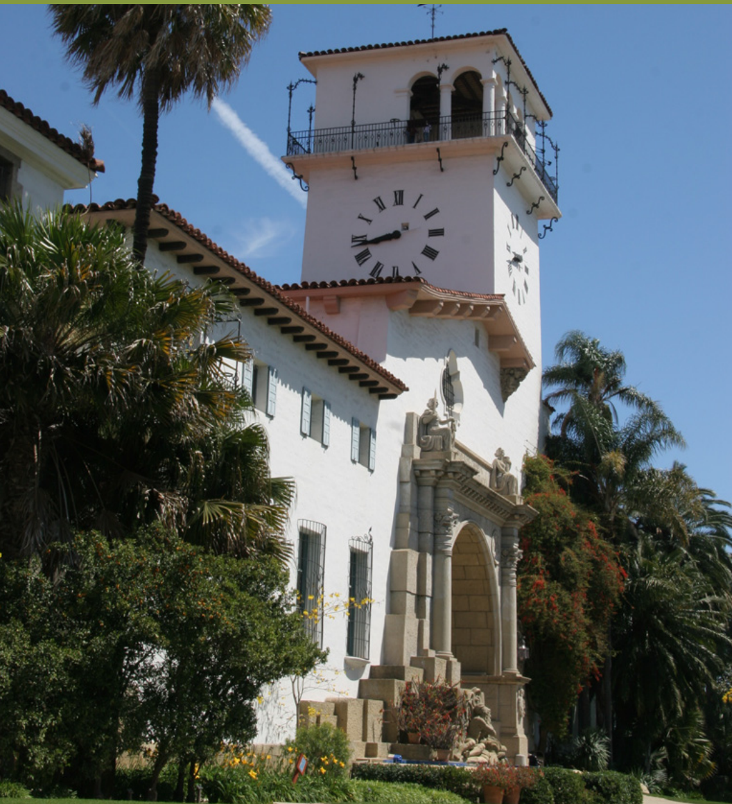
COUNTY COURTHOUSE photo courtesy Robert Ooley
